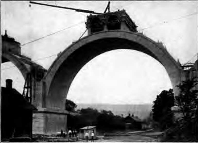
CONCRETE AFFORDS WONDERFUL OPPORTUNITIES FOR THE BRIDGE-BUILDERS
